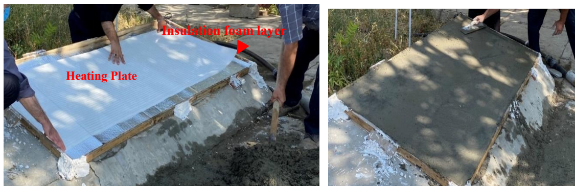
Fig 1 Installation of heating plates on the platform
